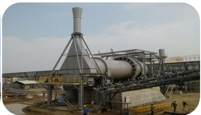
INLET / OULET CHUTE
